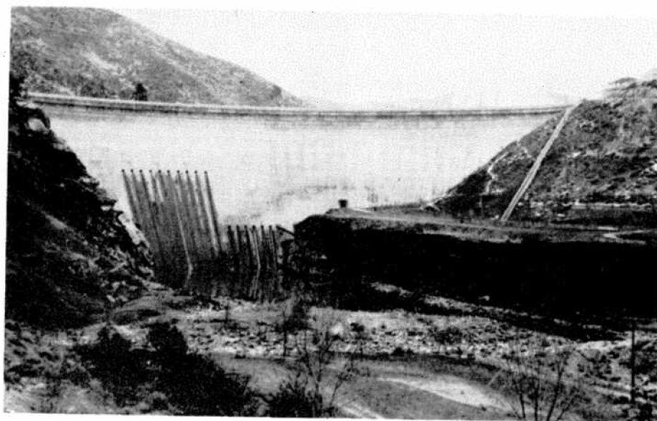
(b) Downstream view
